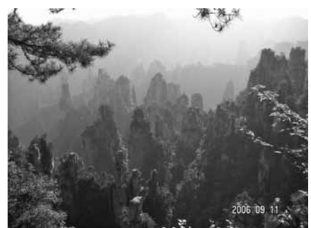
Zhanjiajie is well known for its spectacular scenery. A broadcasting station on top of Tienmenshan with six microwave antennas and an eighty eight meter tower is maintained by fourteen hardworking engineers.
